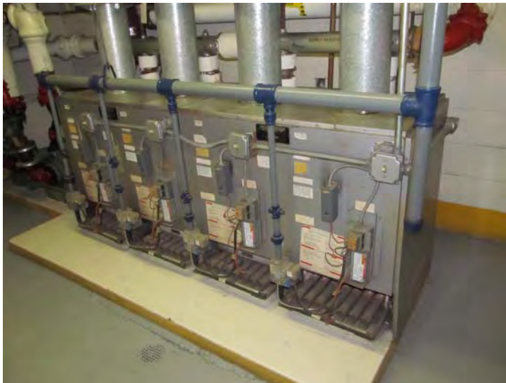
Original Hydrotherm modular boiler plant – No problems observed or reported
