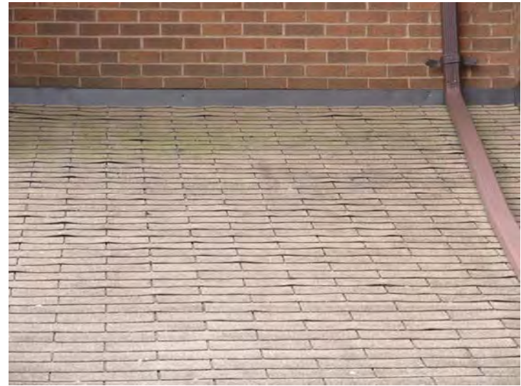
Original roof shingles exhibit signs of age-related wear
