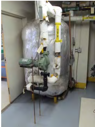
Domestic hot water storage tank with internal heat exchanger
