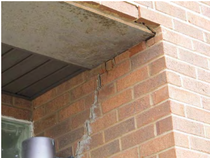
Crack and displacement in brickwork noted at entry to community room on Albany Avenue building elevation
