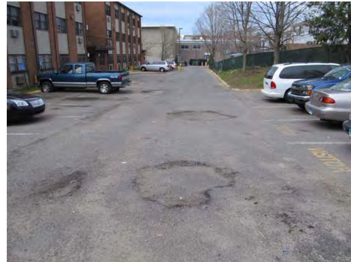
Original asphalt paving in parking area exhibits age-related wear including potholes and cracks
