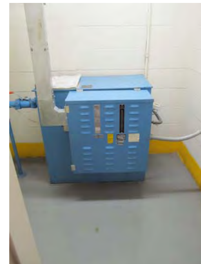
Hydro-mechanical and controller/dispatcher unit for elevator serving all floor levels of building
