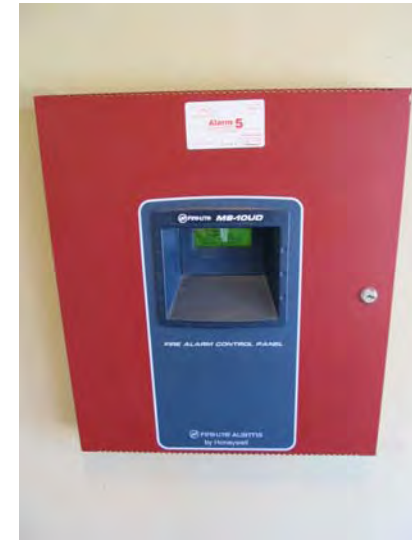
Newer fully addressable fire alarm control panel
