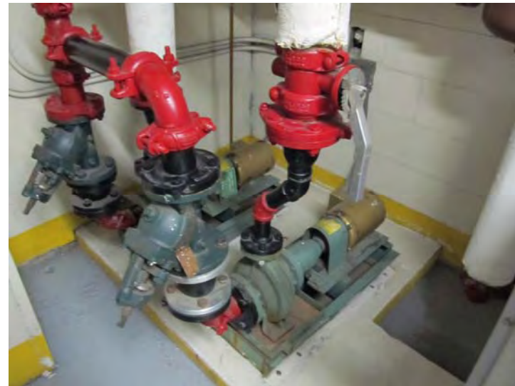
Base-mounted pumps serve to circulate hydronic heat throughout the building
