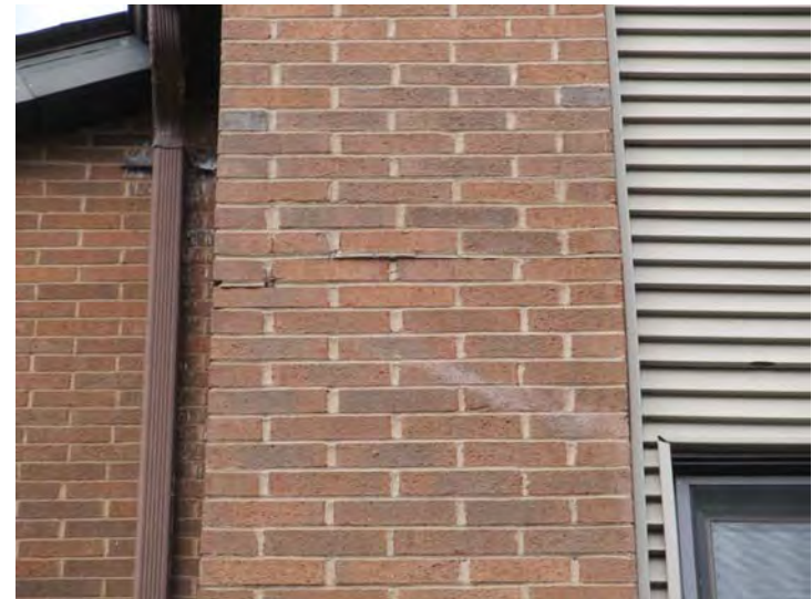
Isolated areas of missing mortar also noted in brickwork
